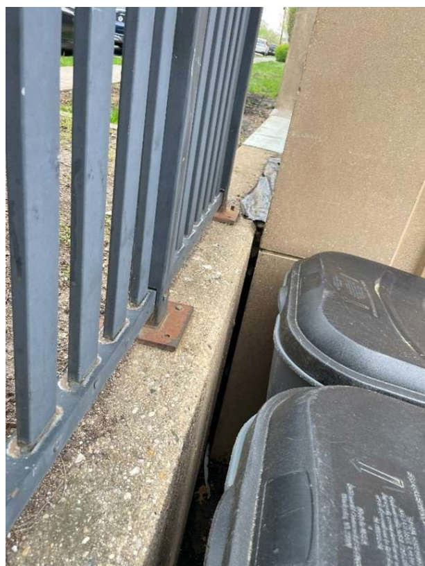
S14 – Railing Fastener Misses
