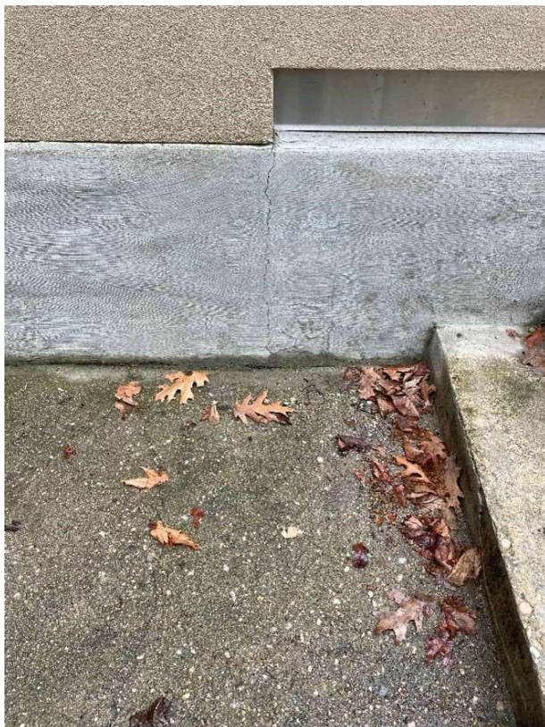
S18 – West Side Foundation Wall Crack
