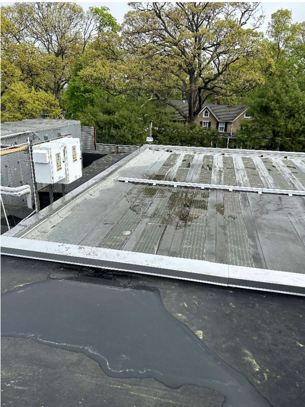
A59 – Ponding at Roof Parapet
