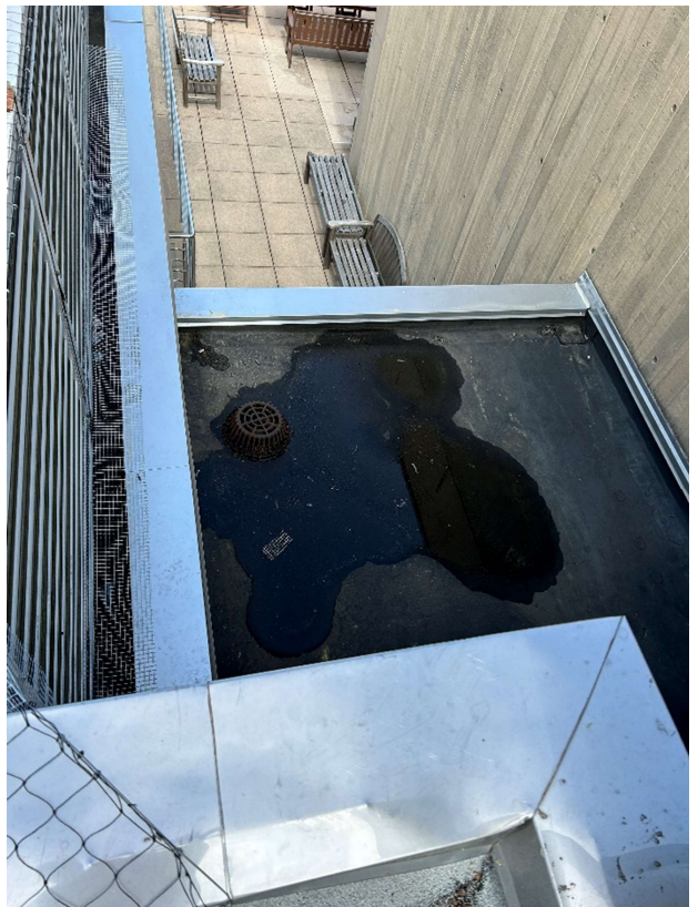
A60 – Ponding at Roof Drain
