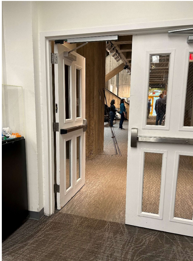
A23 – Computer Lab Fire-rated Door
