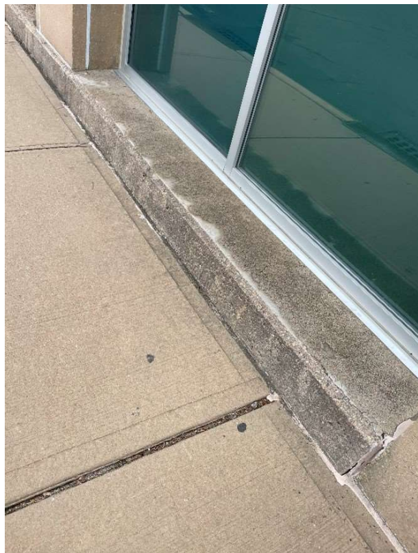
S44 – East Side Foundation Spall
