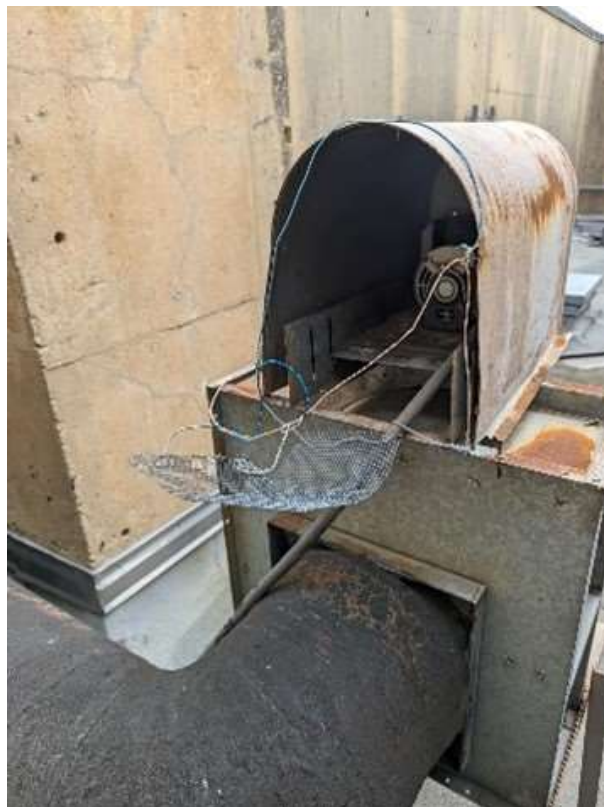
H10 – Typical Exhaust Fan in Poor Condition
