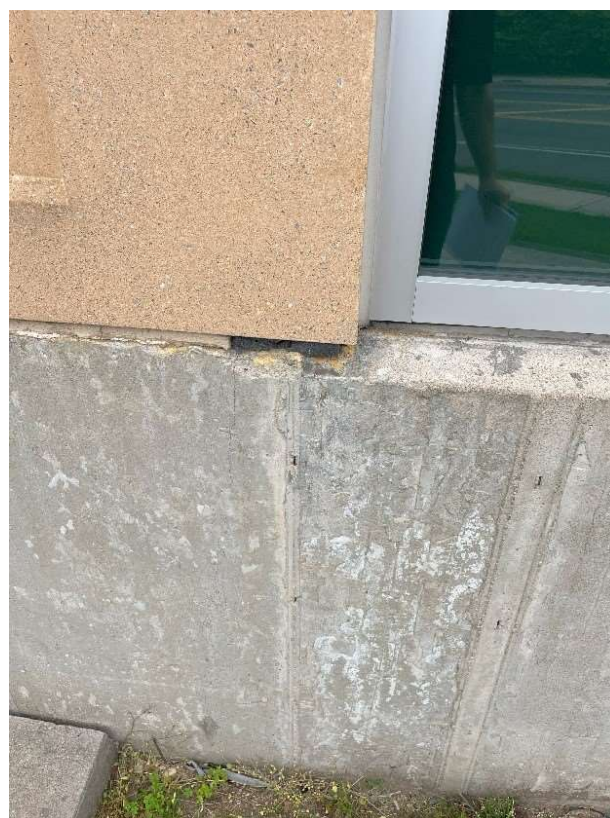
S27 – South Side Sealant Damage
