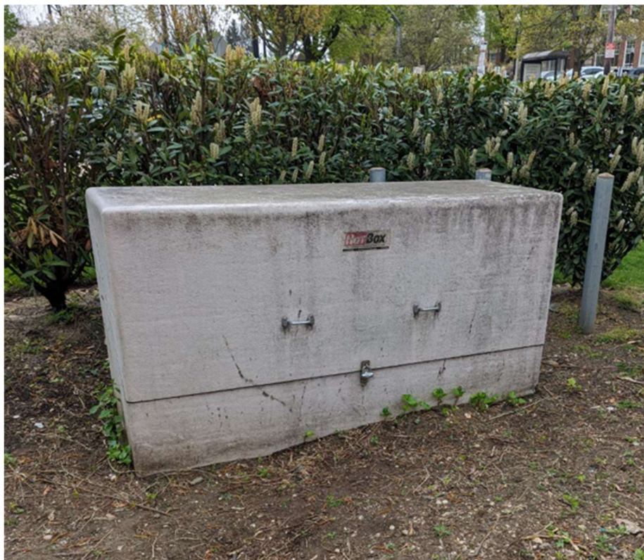
P05 – 2" Domestic Service Heated Enclosure
