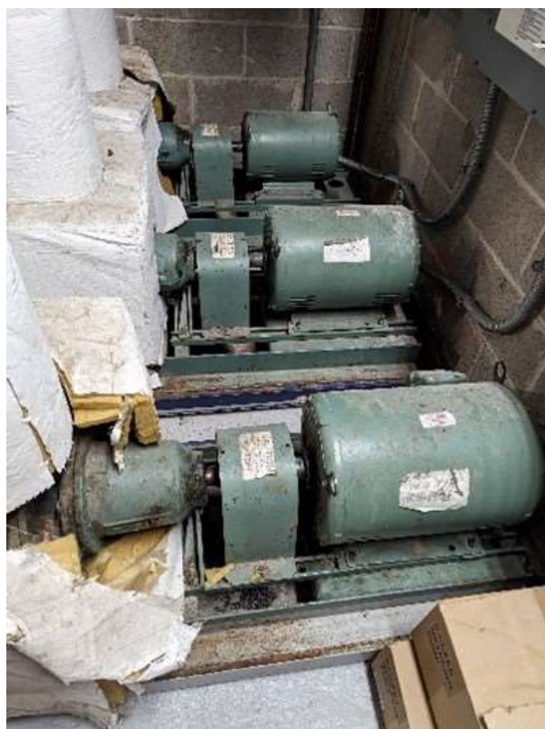
H06 – Chilled & Condenser Water Pumps
