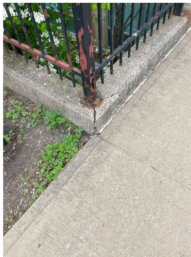
S39 – Railing Corrosion & Spall
