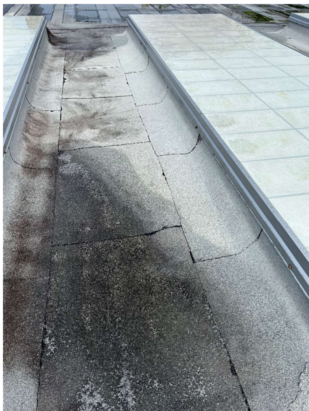
A55 – Roof Membrane Deterioration
