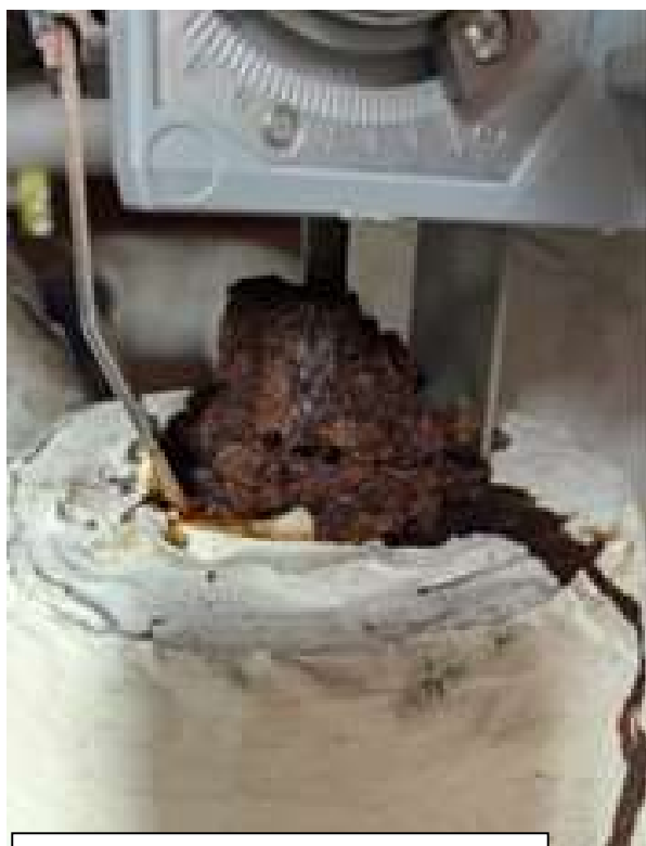
H11 – HVAC Unit Leak
