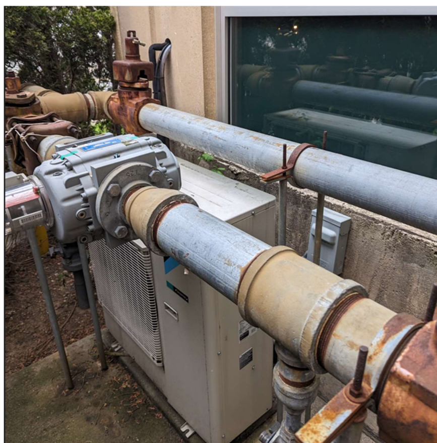
P02 – Gas Meter Rig and Condenser
