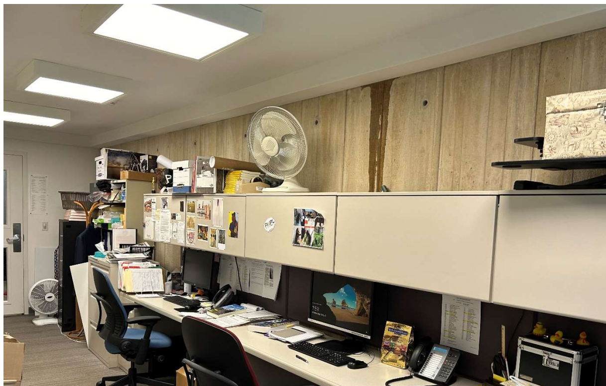
A51 – Leak in Programming Office
