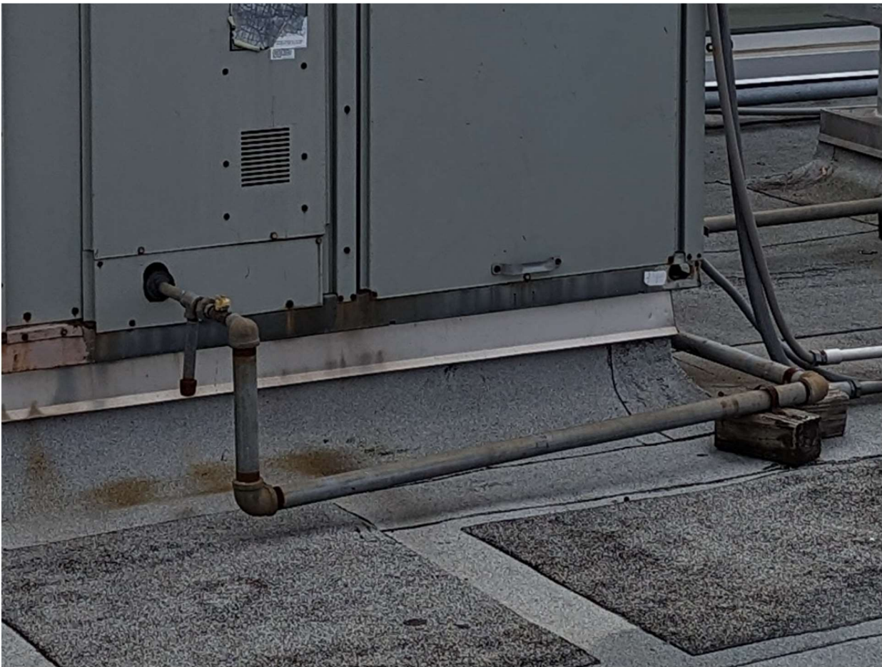
P04 – Rooftop Gas Piping Wood and Inadequate Support
