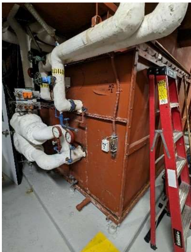
H01 – Typical Multizone Air Conditioner
