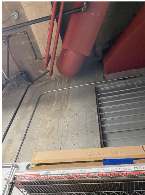
S53 – Evidence of Water Infiltration
