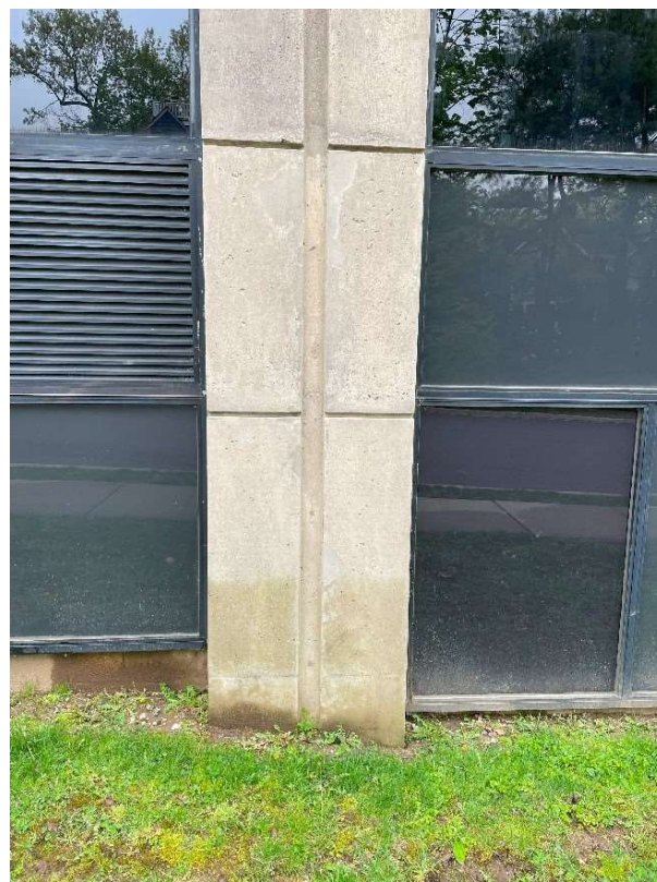
S09 – East Side Honeycombing & Saturation
