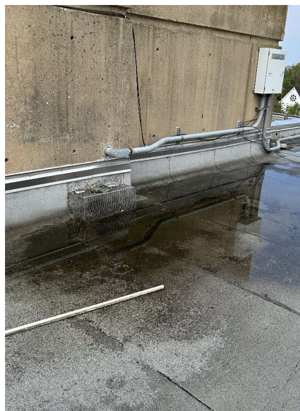
A56 – Ponding at Roof Drain
