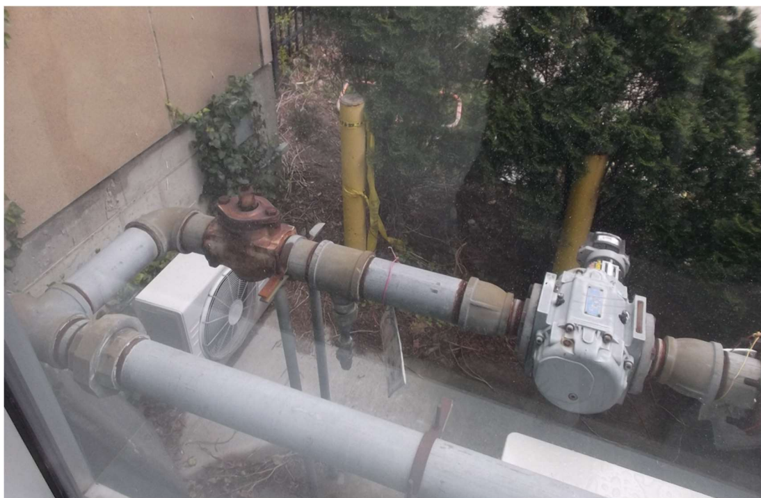
P01 – Gas Meter Rig
