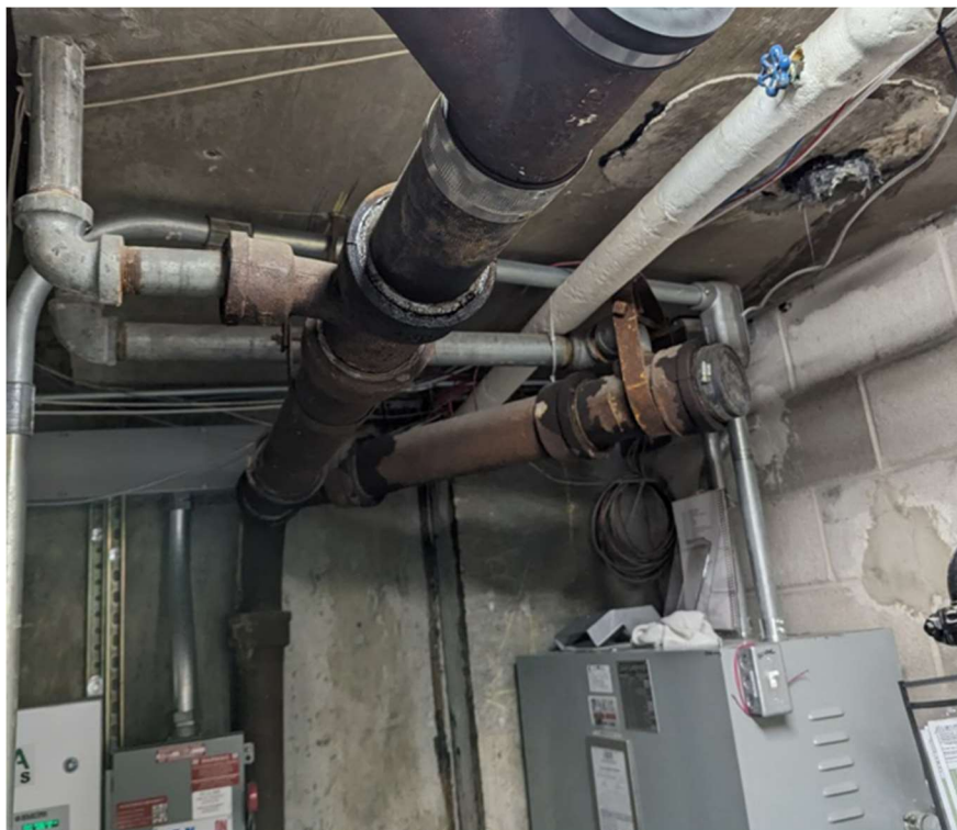
P11 – Pipe above Electrical Equipment
