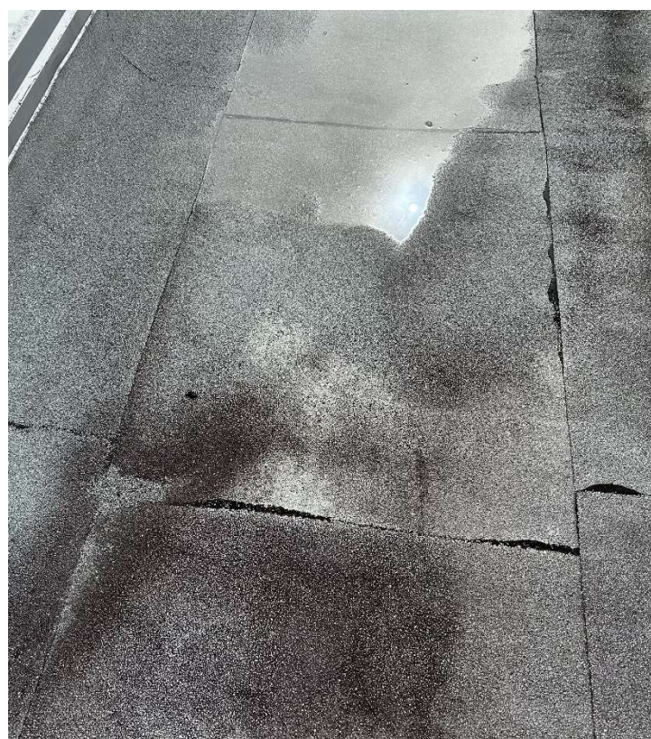
A54– Seams between Roof Membrane
