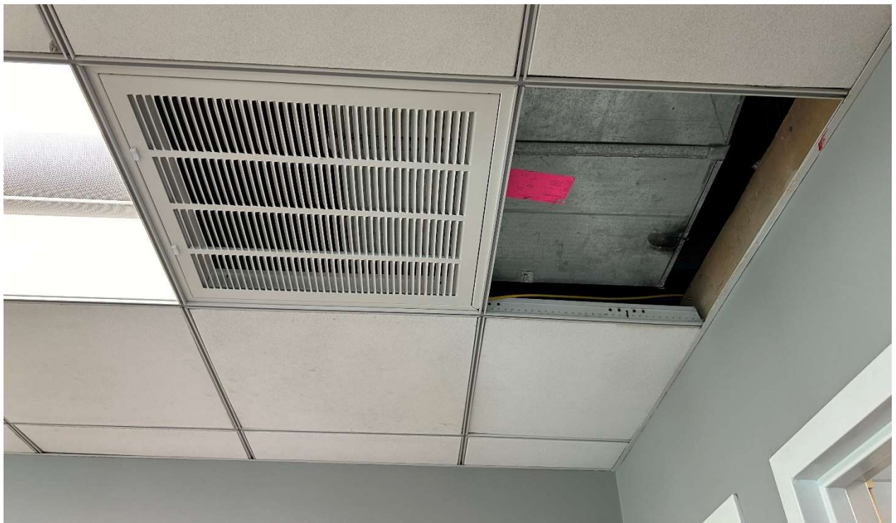
A50 – Leak from Duct
