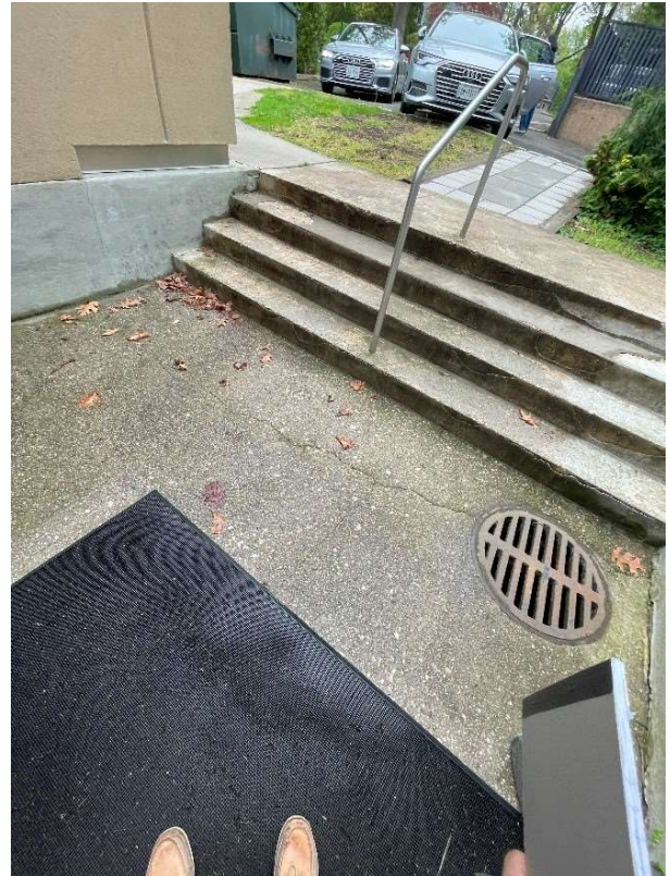
S17 – West Side Step Spall
