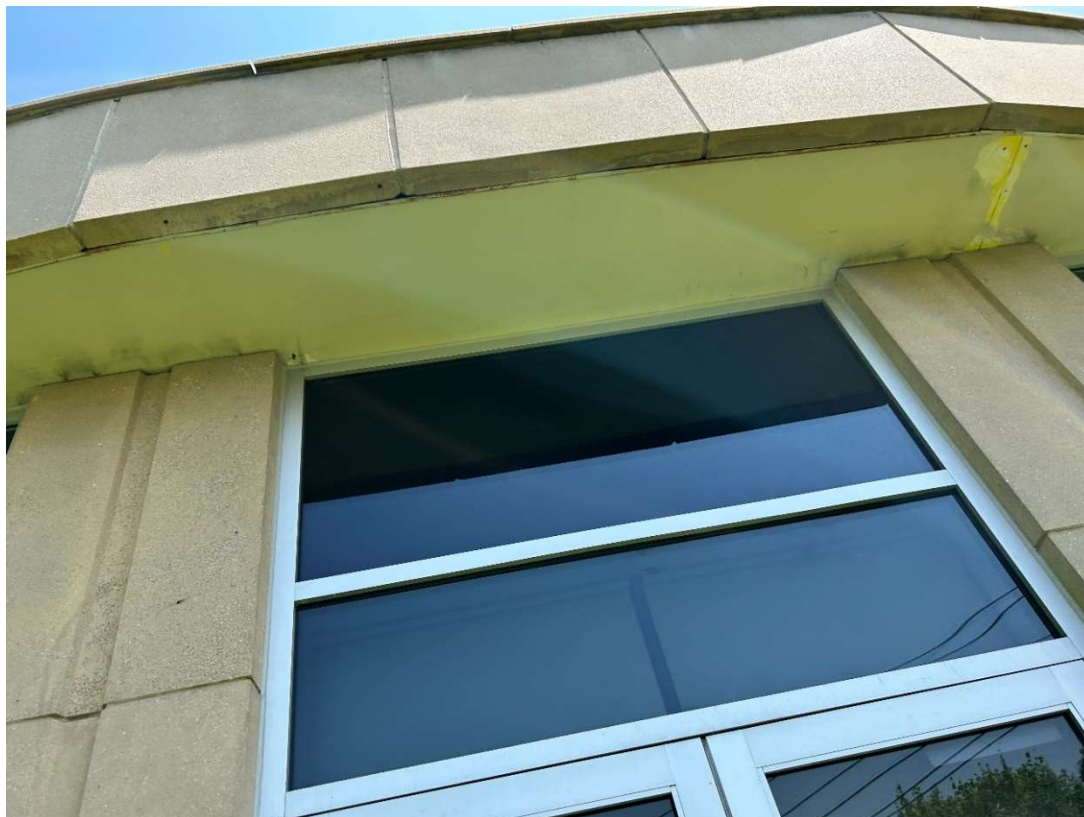
A47 – Terrace Paver Leakage
