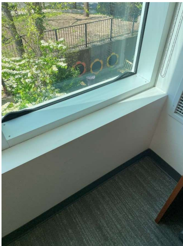
S62 – South Window Seal Failure
