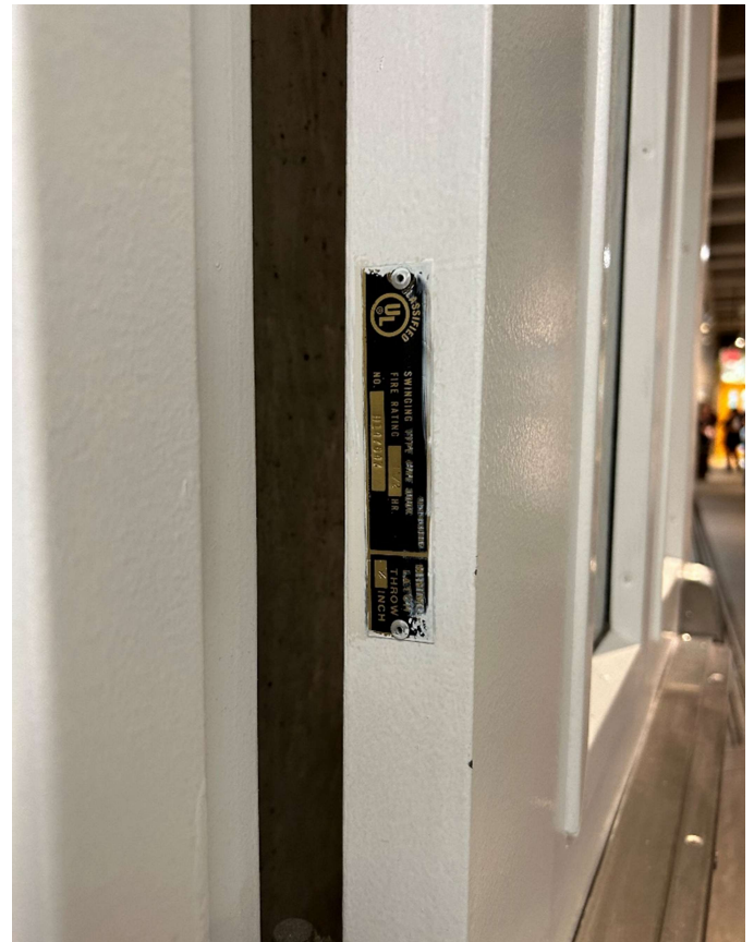
A24 – Computer Lab Fire-rated Door Label
