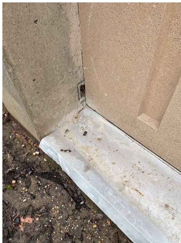
S11 – Exposed Embedded Electrical Box
