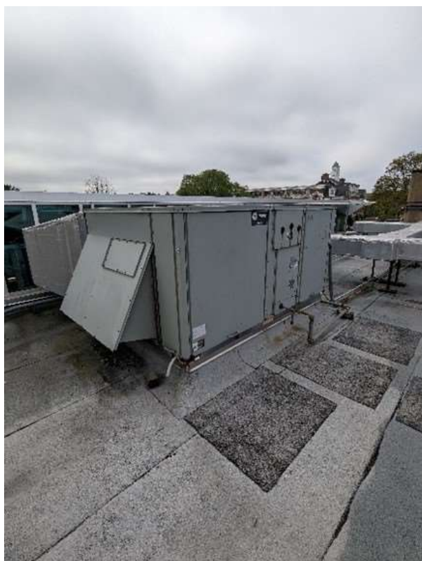
H03 – Typical Packaged Rooftop A/C
