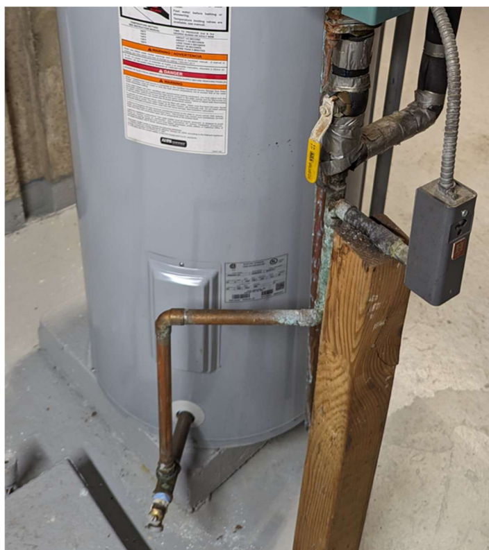
P10 – Water Heater's Corrosion and Wood Support
