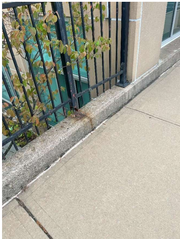
S40 – Railing Corrosion & Crack
