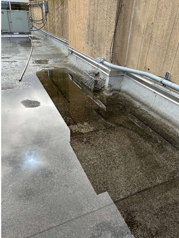
A57 – Ponding at Roof Drain
