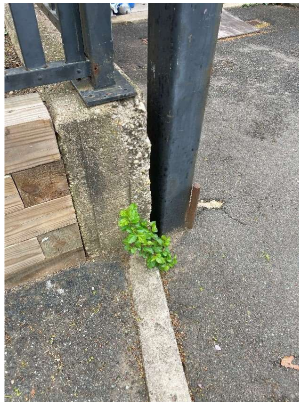
S13 – Spalled Concrete & Fastener Miss
