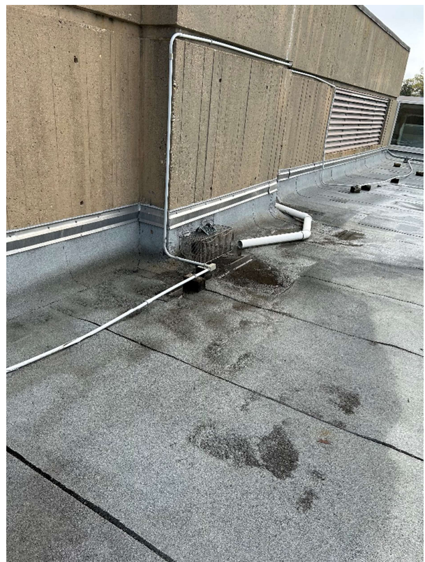
A64 – PVC Conduit on Roof
