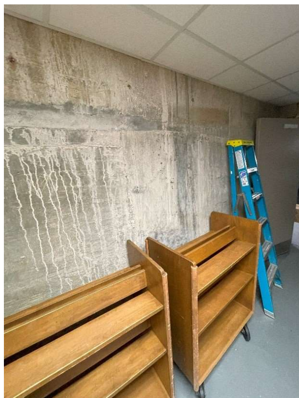
S54 – Basement Foundation Cracking
