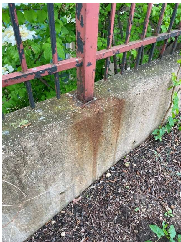
S38 – Railing Corrosion & Crack
