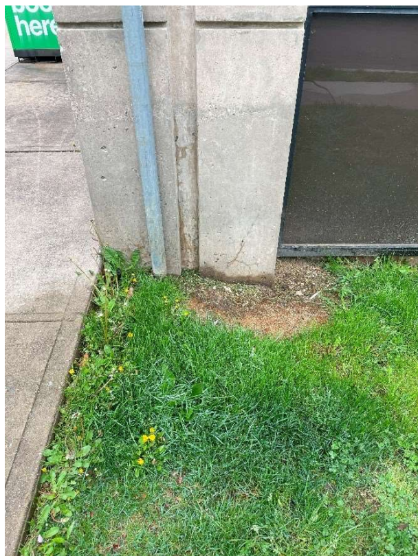
S08 – East Side Corner Cracking & Saturation
