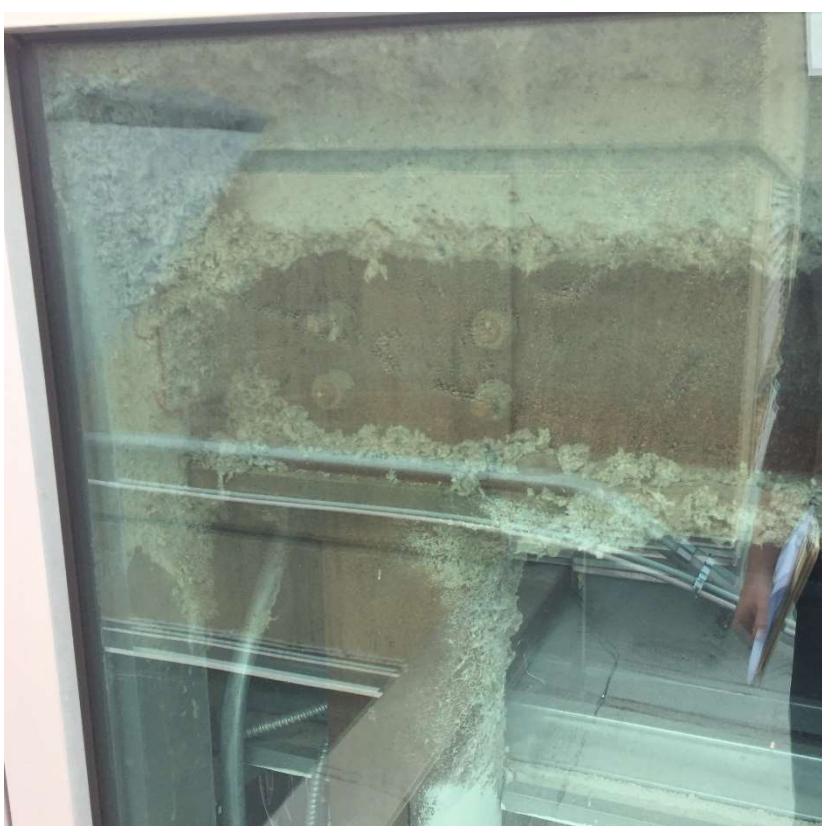
A68 – Fireproofing Deterioration
