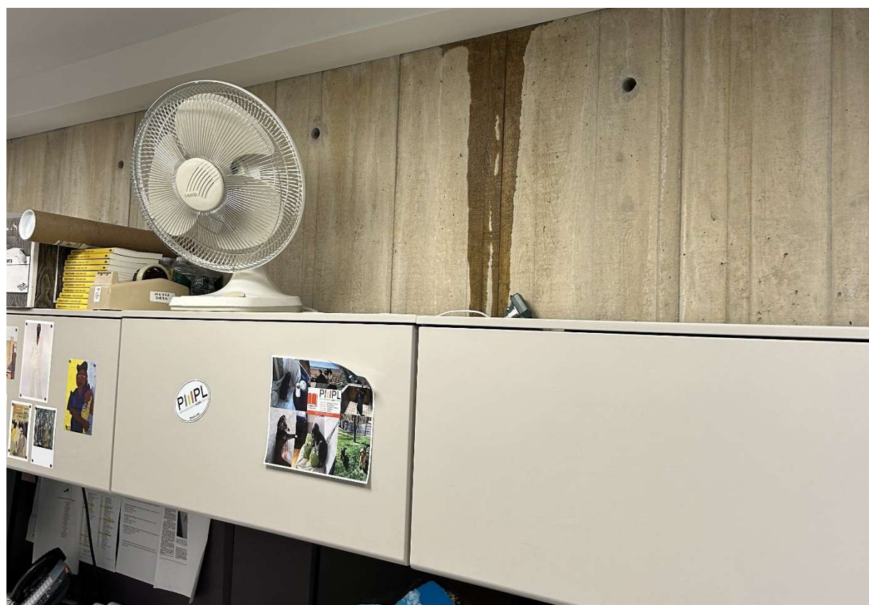
A52 – Leak in Programming Office
