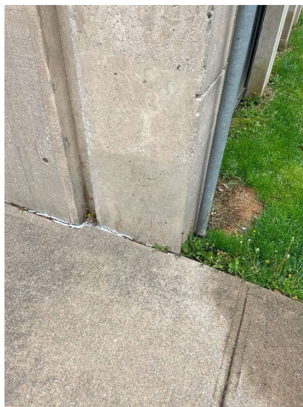
S07 – East Side Corner Cracking
