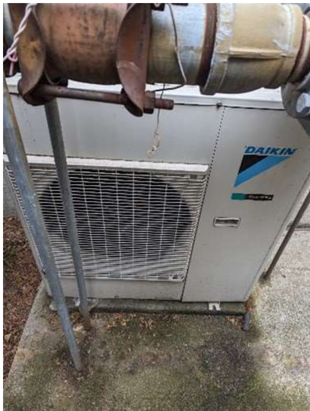
H09 – Typical Ductless Split Condensing Unit
