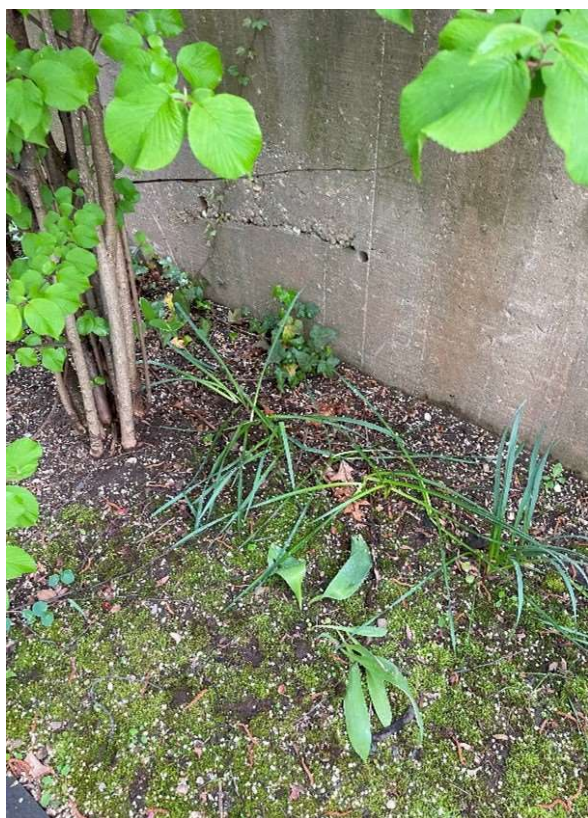
S34 – Retaining Wall Honeycomb / Crack
