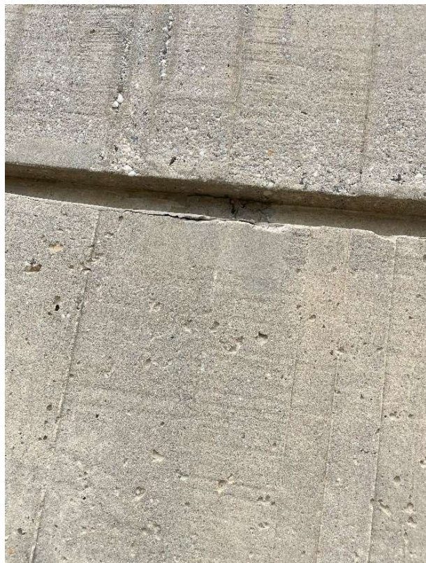
S04 – East Side Spall
