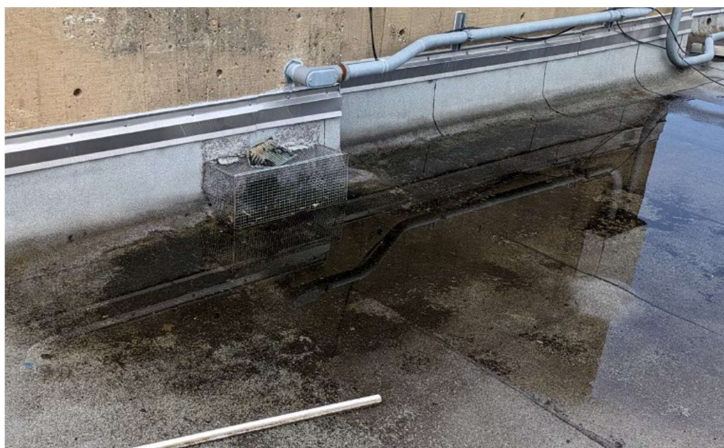
P14 – Ponding of Roof
